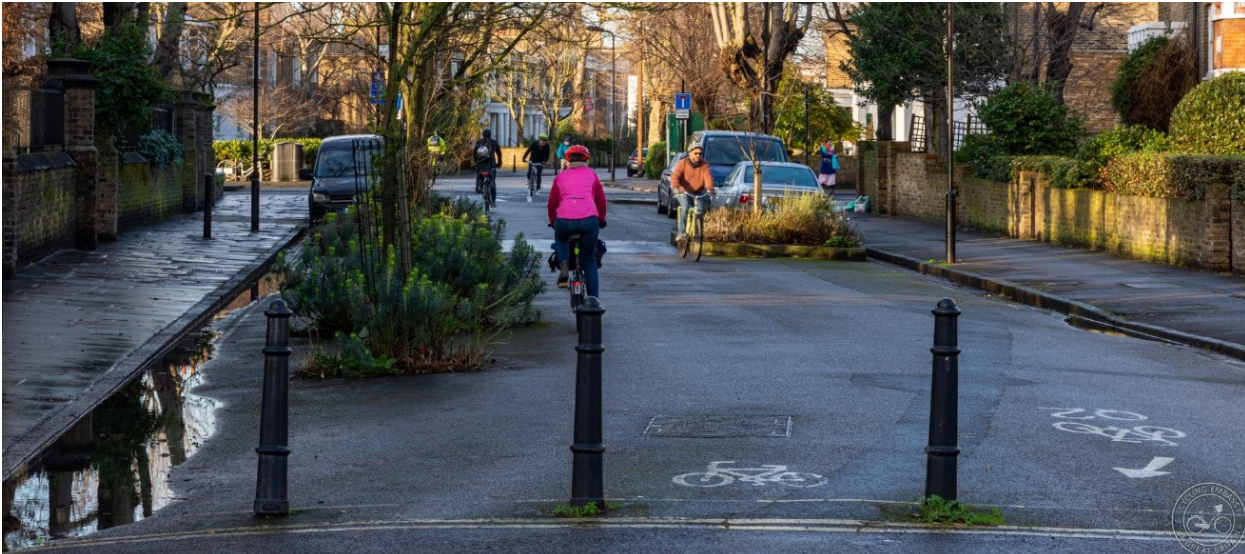
Bollards acting as a modal filter, limiting through-traffic to pedestrians and cyclists only. Source: Cycling Embassy of Great Britain
