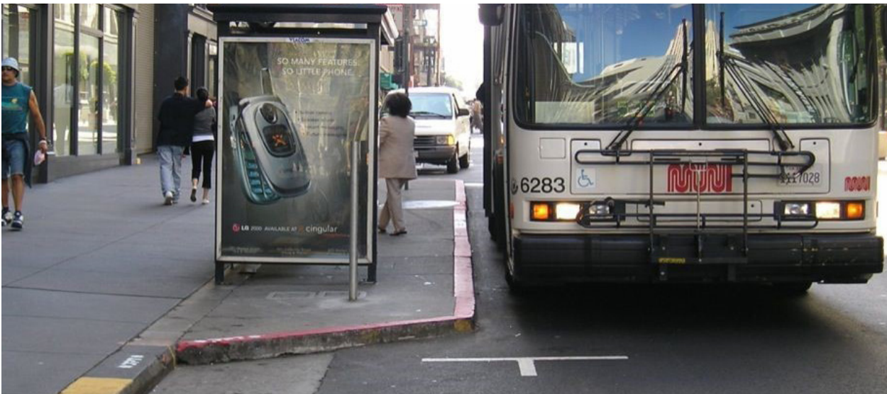
Shared space bus stop on a curb bump out in San Francisco. Source: NACTO
