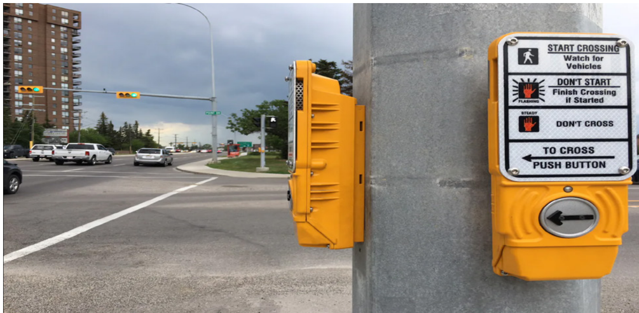
Accessible pedestrian signals help those with visual or auditory disabilities safely cross the street. Source: CBC
