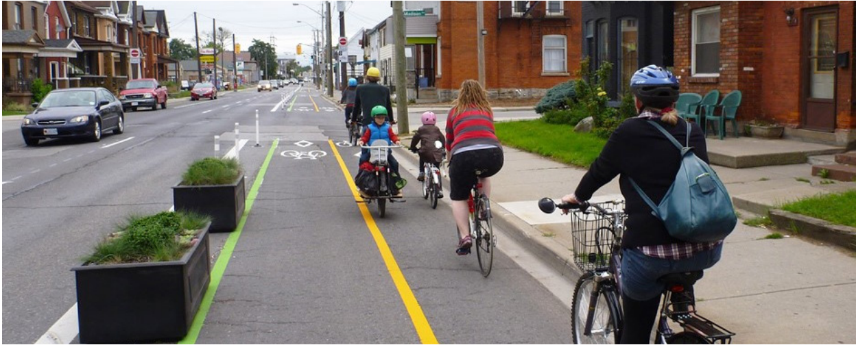
This cycle track in Hamilton uses planters to separate cyclists from vehicle traffic. Source: Canadian Consulting Engineer
