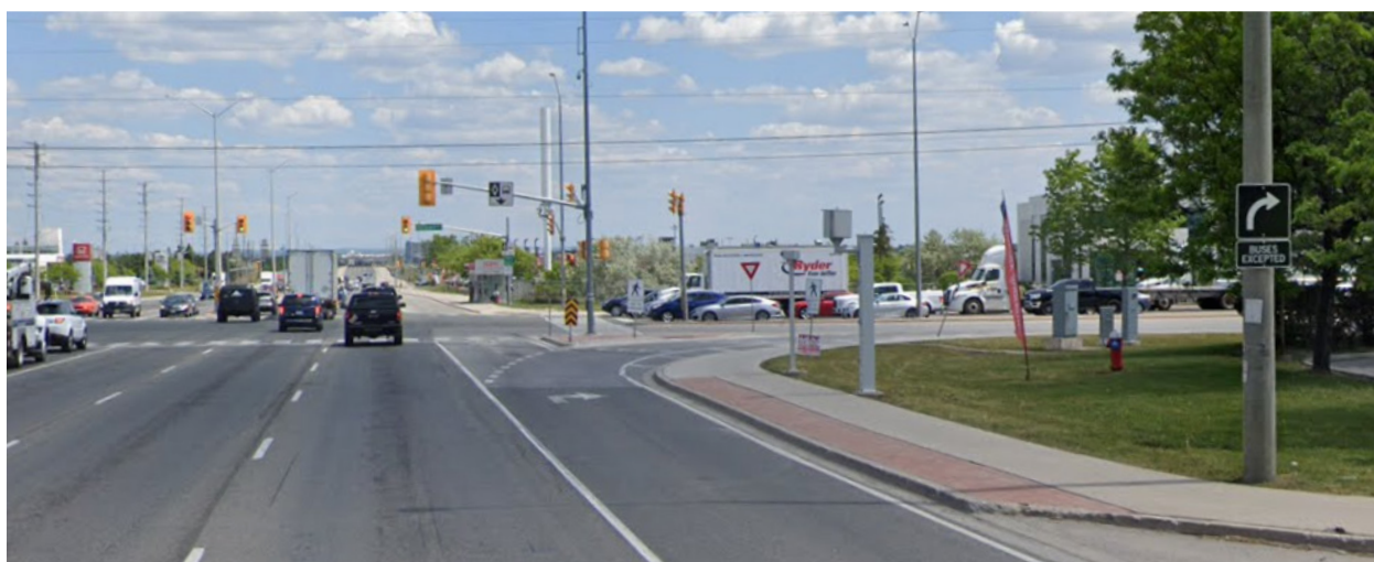
Right-turn lane used as a queue jump lane for buses in Brampton, ON. Source: Google maps
