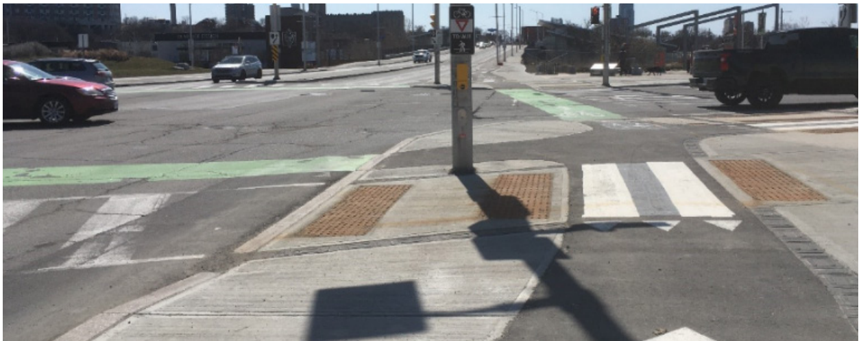
An example of a pedestrian refuge between a cycle track and roadway crossing, denoted by attention TWSI's at each end. Ottawa, ON
