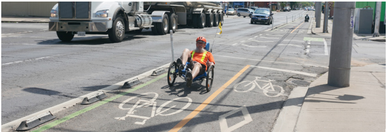
It is important to consider a variety of users and their levels of accessibility when designing for Complete Streets.
