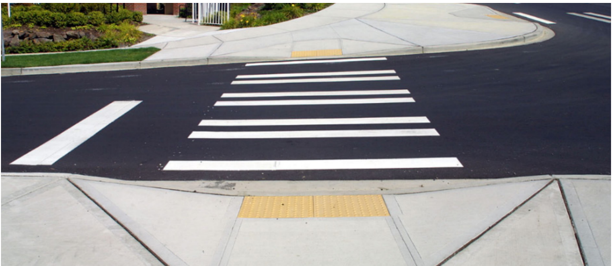
Example of a depressed curb ramp at a pedestrian crossing in Washington State. Source: Pedestrian Safety Guide and Countermeasure Selection System
