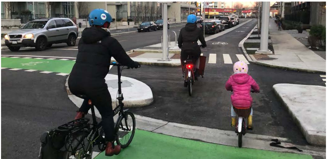
A protected intersection where cyclists are protected from vehicle traffic via a setback intersection crossing, curbs, and brightly coloured bike lanes. Source: NACTO
