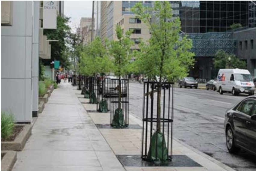
Continuous growing trench in streetscape. Source: Draft Design and Preservation Standards for Public Property
