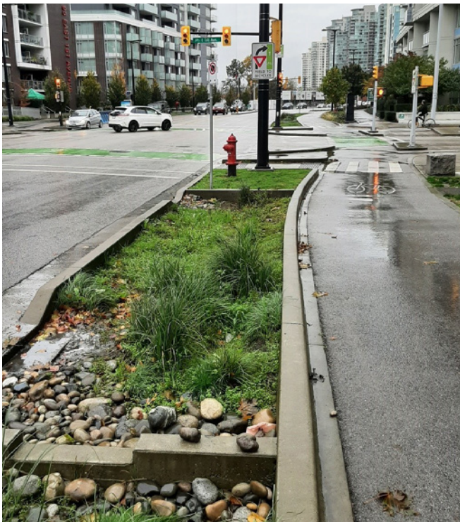
Low impact development feature separating a protected bike lane from automobile traffic, in Vancouver, BC
