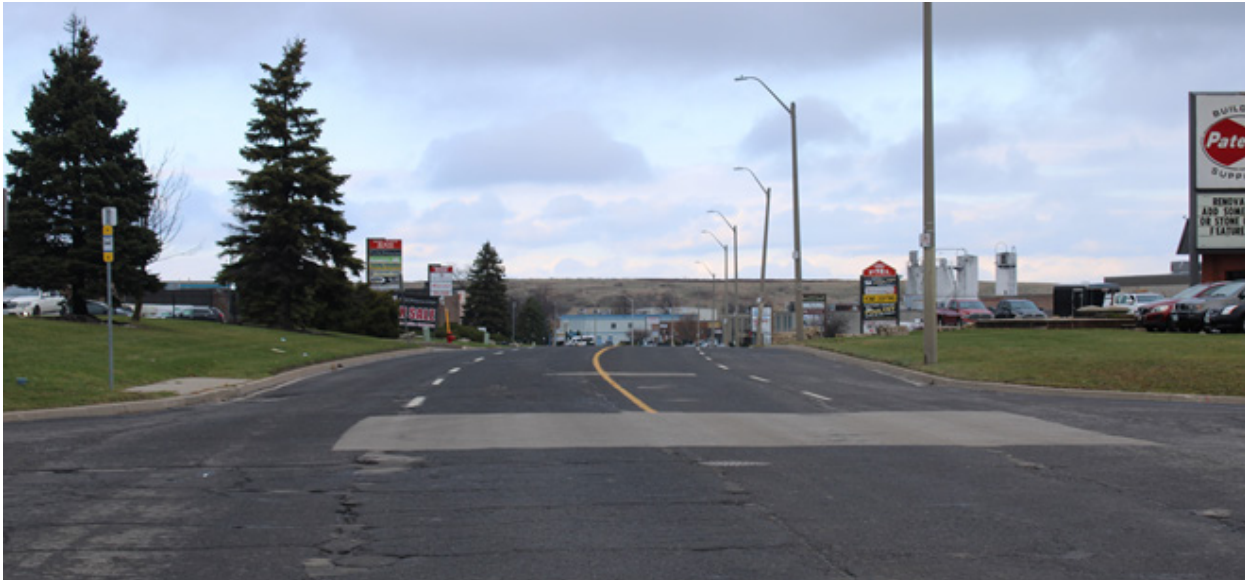
Nebo Road at Lansing. Source: Google Maps
